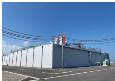
Wastewater treatment facility in Oita Plant
