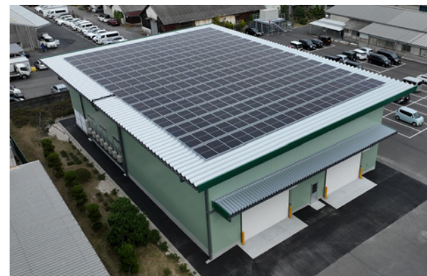
Overhead view of warehouse enlisting Net ZEB design
