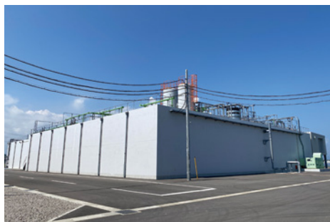
Wastewater treatment facility in Oita Plant
